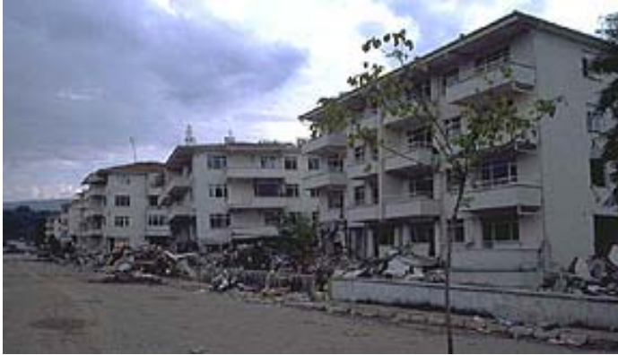
Figure 3-12 Collapse of moment frame buildings, Gölcük
