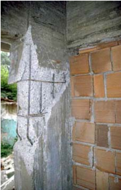
Figure 3 –26 Typical transverse reinforcement details in columns a. view of damaged blade column b. transverse tie details in blade column
