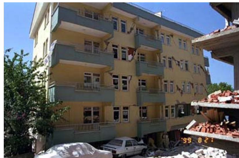
a. Collapsed building
