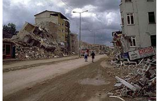
Figure 3-13 Collapse of moment-frame and wall buildings, Adapazari
