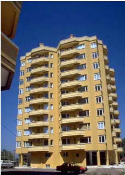
Figure 3-1 High quality apartment construction, Yalova
