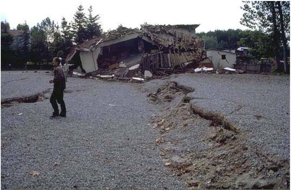
Figure 3-14 Collapsed school building that straddled the line of rupture
