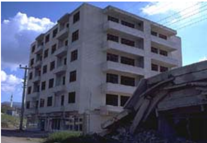
a. lightly damaged six-story building
