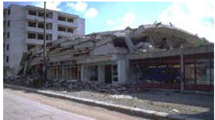
b. collapsed six-story building
