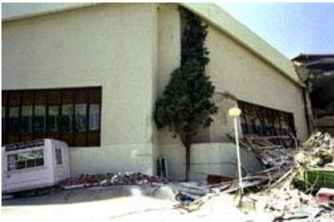
Figure 3-40 a. Shear wall building damaged due to fault rupture
