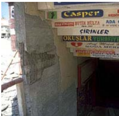
Figure 3-43 Damage to short wall / blade column
