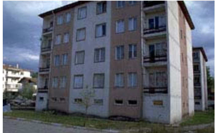
Figure 3-39 Undamaged apartment building in Gölcük
