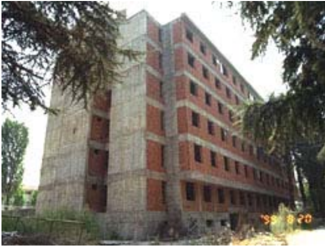
Figure 3-38 Shear wall building under construction at the time of the earthquake
