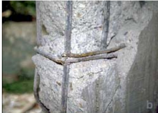
Figure 3 –26 Typical transverse reinforcement details in columns a. view of damaged blade column b. transverse tie details in blade column
