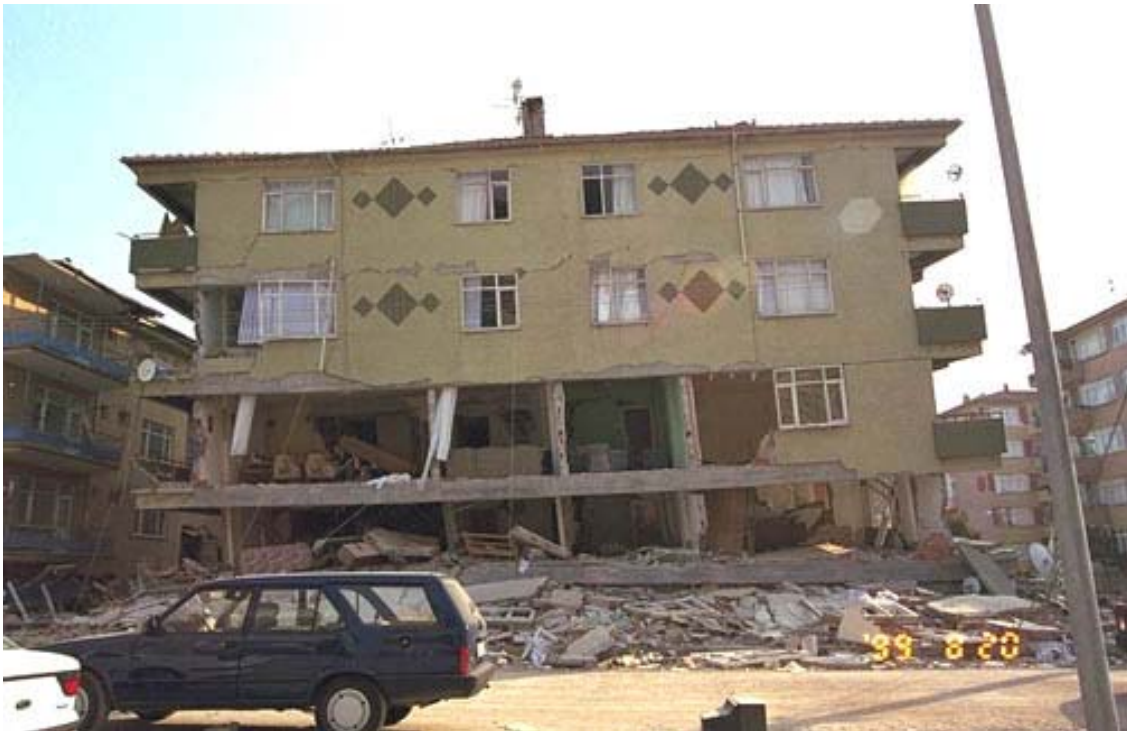
Figure 3-22 Failure of two stories of moment-frame building with infill masonry
