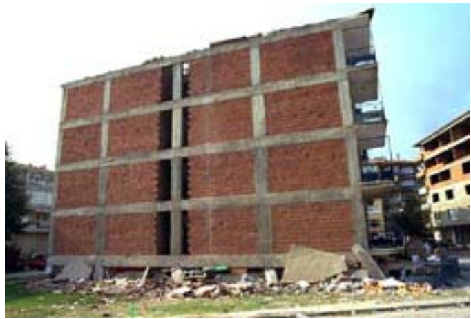
b. view of infill wall perpendicular to sidewalk
