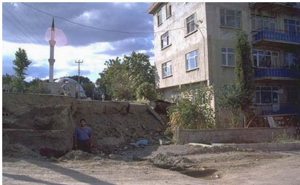
Figure 3-17 Undamaged building located within 2 m of the line of rupture
