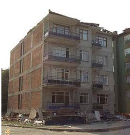
a. view of front face of building
