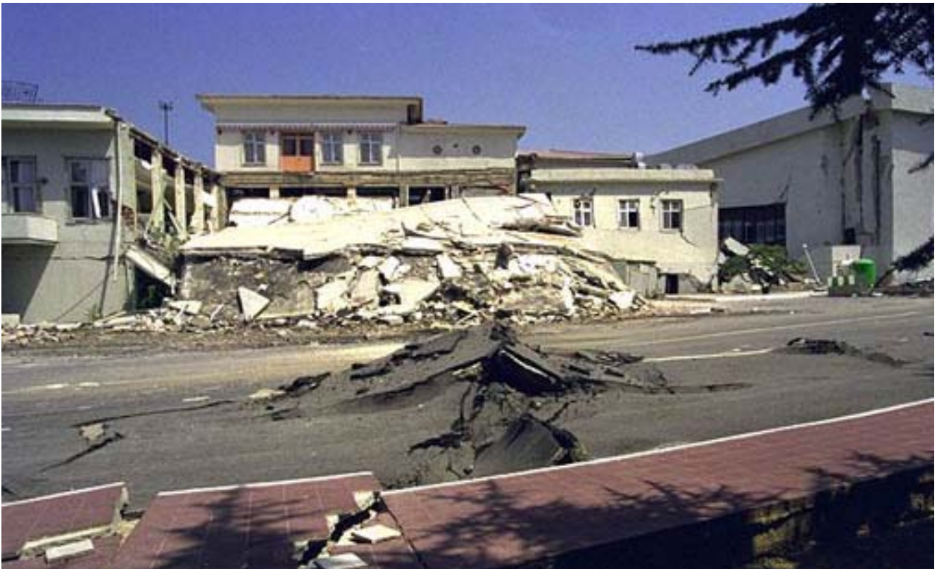
Figure 3-15 Collapsed and damaged moment-frame buildings on the Gölcük navy base
