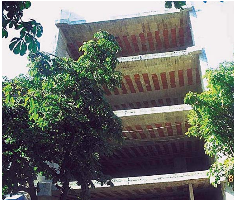
Figure 3-11 Asmolen floor system in a four-story building
