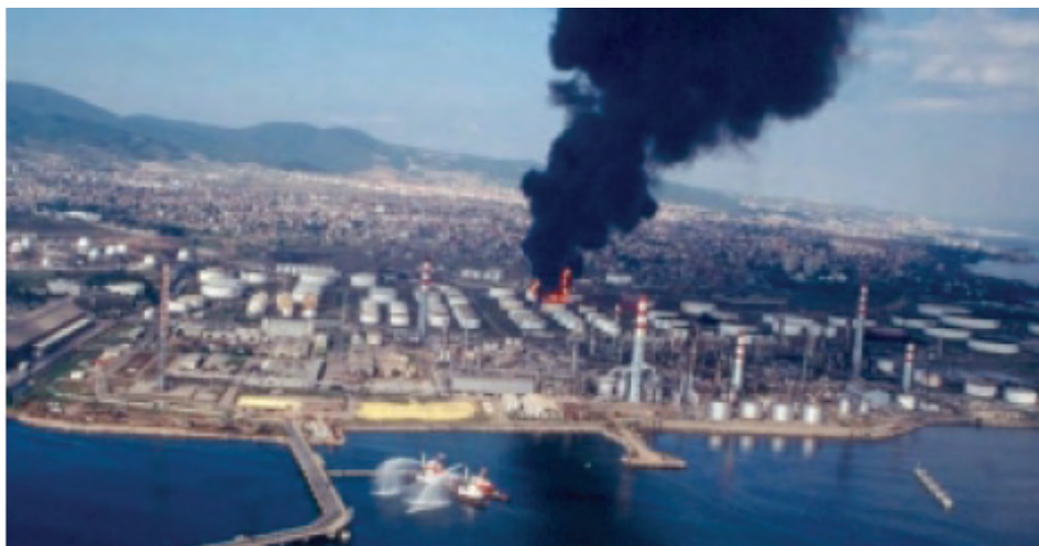
Fig. 2. A view of the fire in TUPRAS petrochemical complex (Erdik, 2007)
