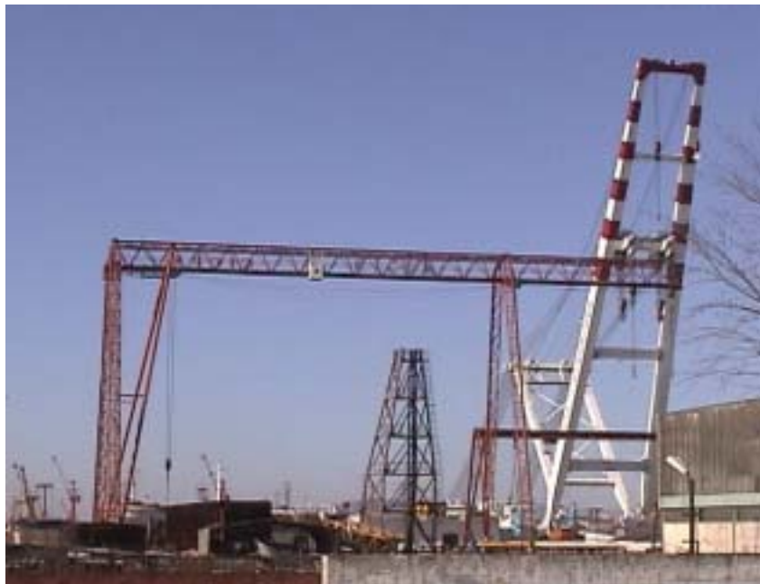
Figure 3.2.74. A large crane in Tuzla Dockyard
