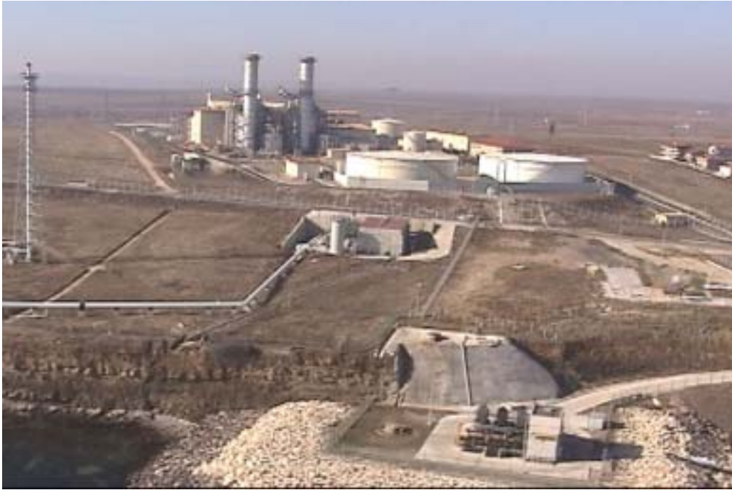
Figure 3.2.92. LNG Power Station No:1 in Marmara Ereğlisi which is being operated by the company ENRON..
