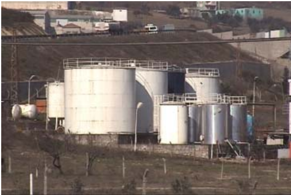
Figure 3.2.44. The storage tanks in northern Dilovasi
