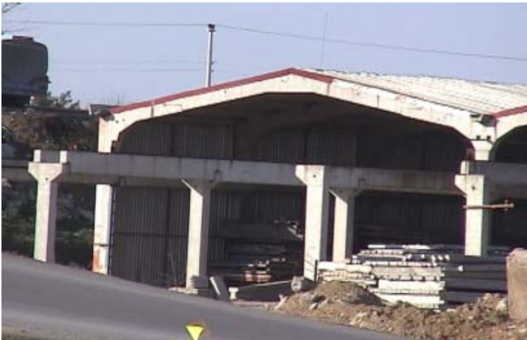
Figure 3.2.63. Typical Prefabricated (PF) building structure in Gebze, (under construction).
