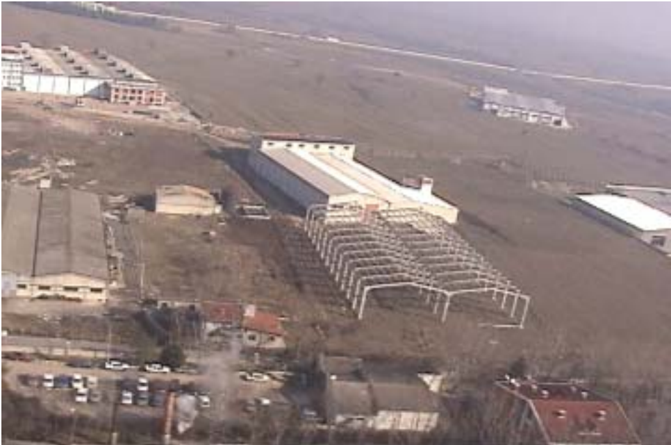
Figure 3.2.99. Typical construction type for the industrial facilities near Cerkezkoy
