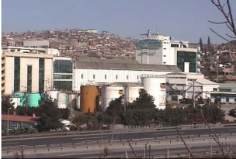
Figure 3.2.30. Storage tanks of a paint production factory.
