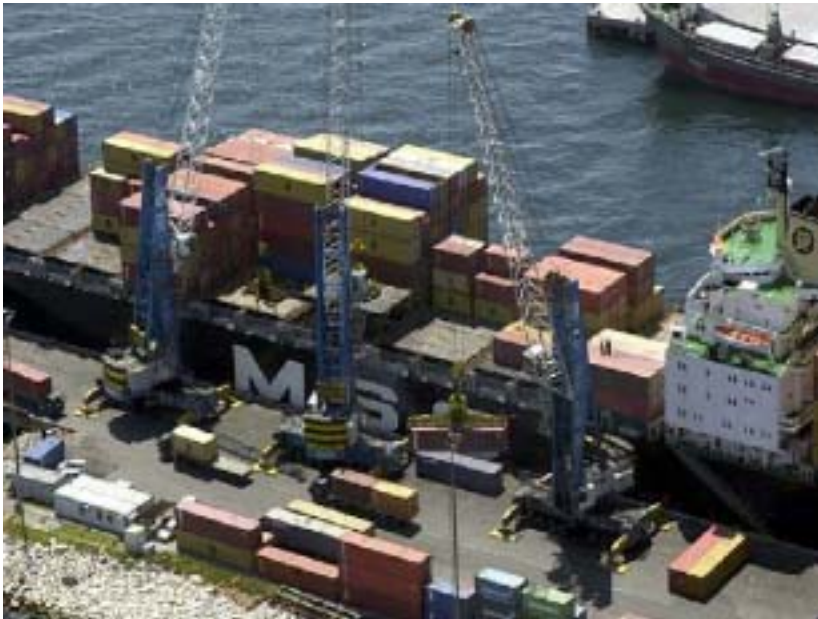
Figure 3.2.86. The winches, containers and cargo equipments in Region 2
