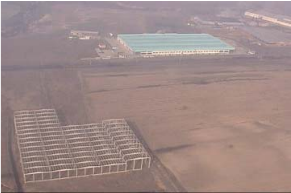
Figure 3.2.98. Construction of a prefabricated structure on a wide area in Cerkezkoy.
