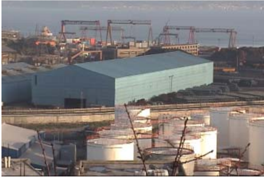
Figure 3.2.26. Typical building structures, storage tanks and cranes in southern Dilovası.
