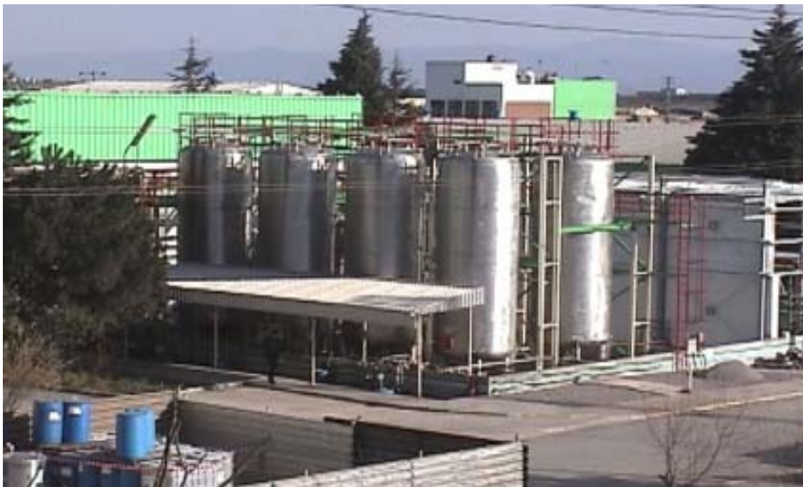
Figure.3.2.65. The storage tanks of the Bayer company chemical plant, located on the E-5 Highway, in Gebze.
