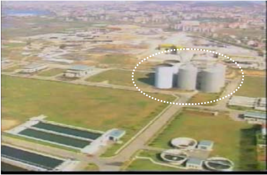
Figure 3.2.77. General view of the waste water treatment plant site in Tuzla, aerial photo.
