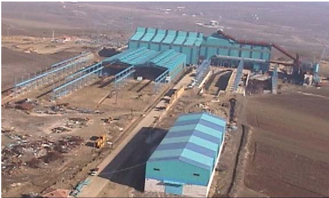
Figure 3.2.95. A steel structure under construction near Botas company in Marmara Ereğlisi.
