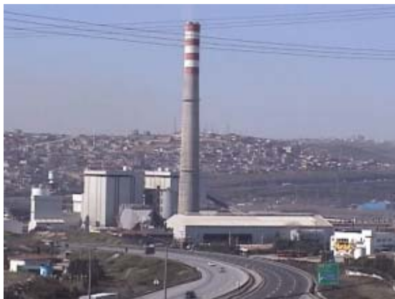
Figure 3.2.29. The 175 meters tall R/C chimney of a paint production factory in central Dilovası.
