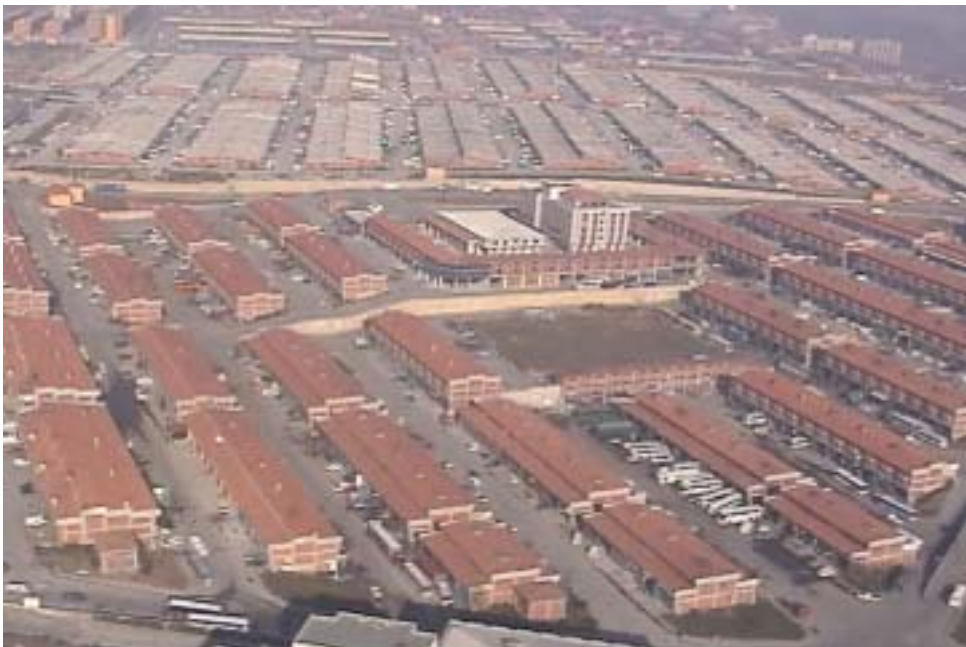
Figure 3.2.103. Aerial view of the industrial park in İkitelli.
