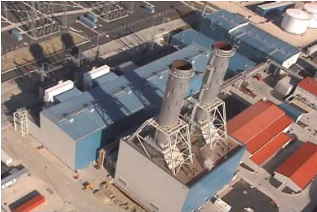
Figure 3.2.93. The electrical equipments of the Power station No:1
