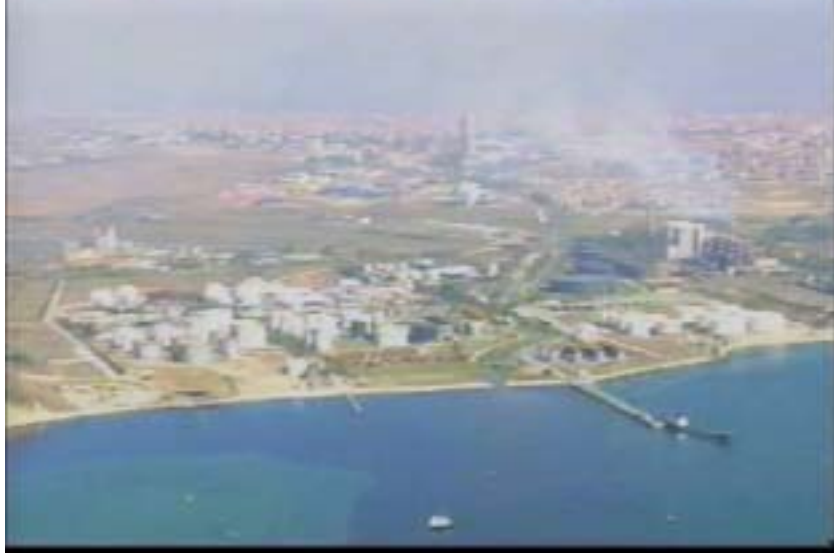
Figure 3.2.84. Aerial view of the Region 1 (Oil platforms and Buoys) of the Ambarli Port
