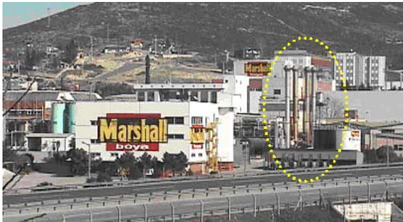
Figure 3.2.31. Tall and slender steel storage tanks of the paint production factory.
