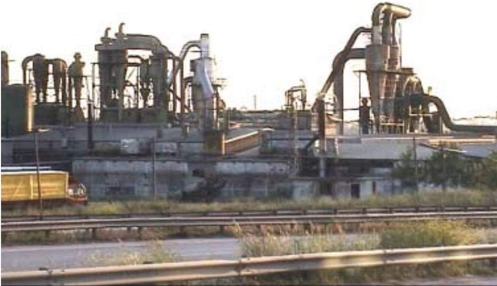
Figure 3.2.60. An industrial facility for drying wood shavings.
