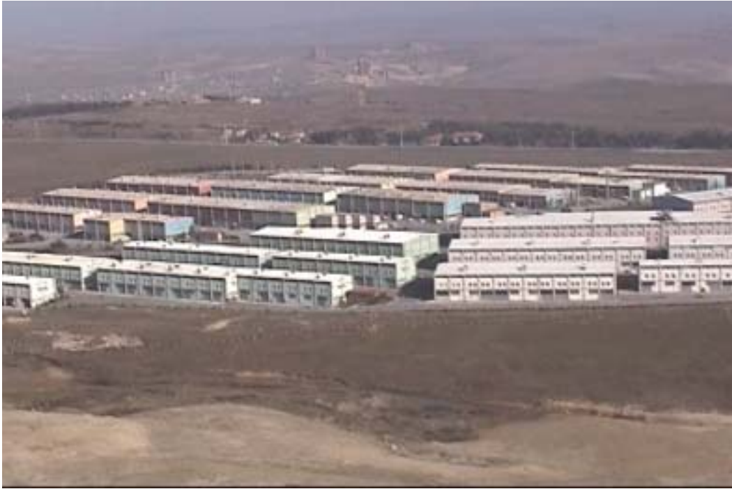
Figure 3.2.102. A typical industrial park consisting of small to medium size P.F. facilities near Catalca
