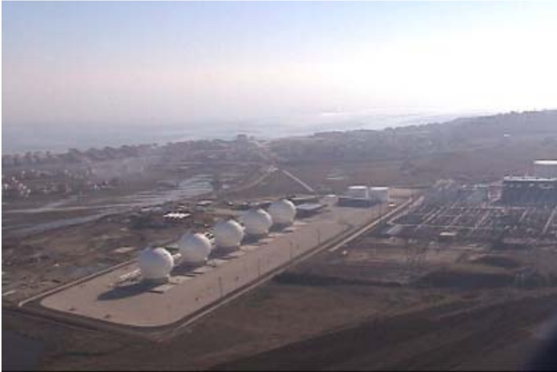
Figure 3.2.94. The LPG storage tanks in Marmara Ereğlisi, near Botas.
