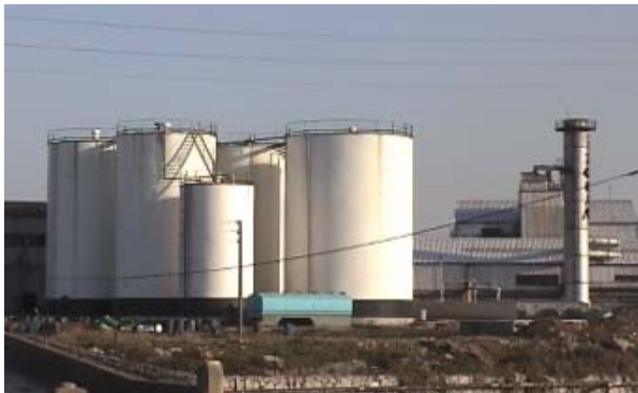
Figure 3.2.40. Vertical storage tanks in central Dilovasi
