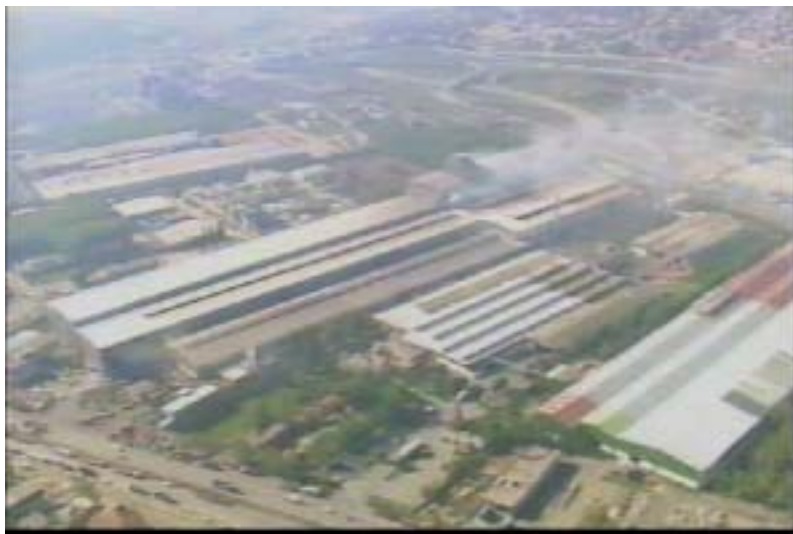
Figure 3.2.32. Steel mills in central Dilovası , (from north.)
