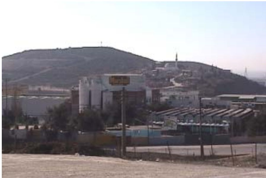
Figure 3.2.36. Vertical storage tanks of Marshall paint factory.
