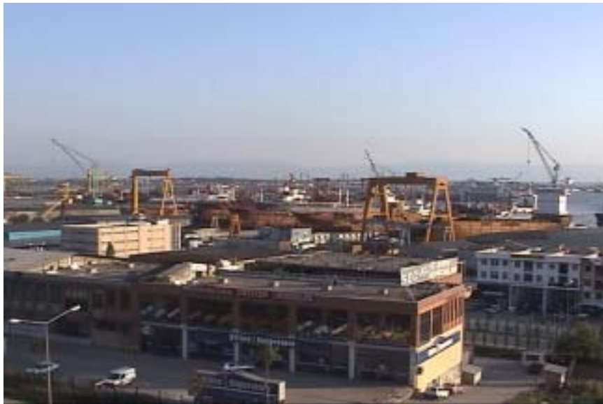
Figure 3.2.69. General view of the Tuzla Dockyard, (from north)
