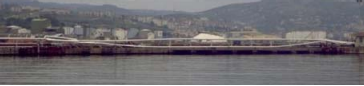
Figure 4.25. Settlement at Petrol Ofisi pier.
