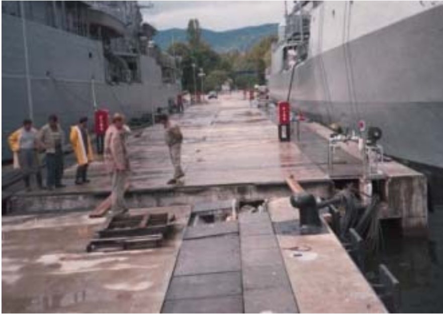
Figure 4.20. Fault offset on the navy port at Golcük.
