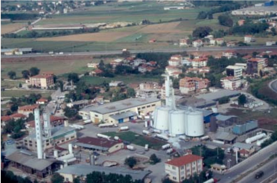
Figure 4.30. Damage at Habaş Facility.
