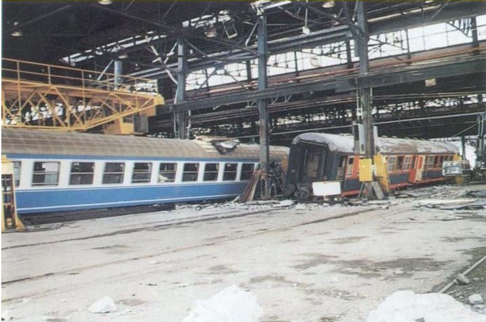
Figure 4.36. Damage at TUVASAŞ Rail Car Factory (after Milli-Re).
