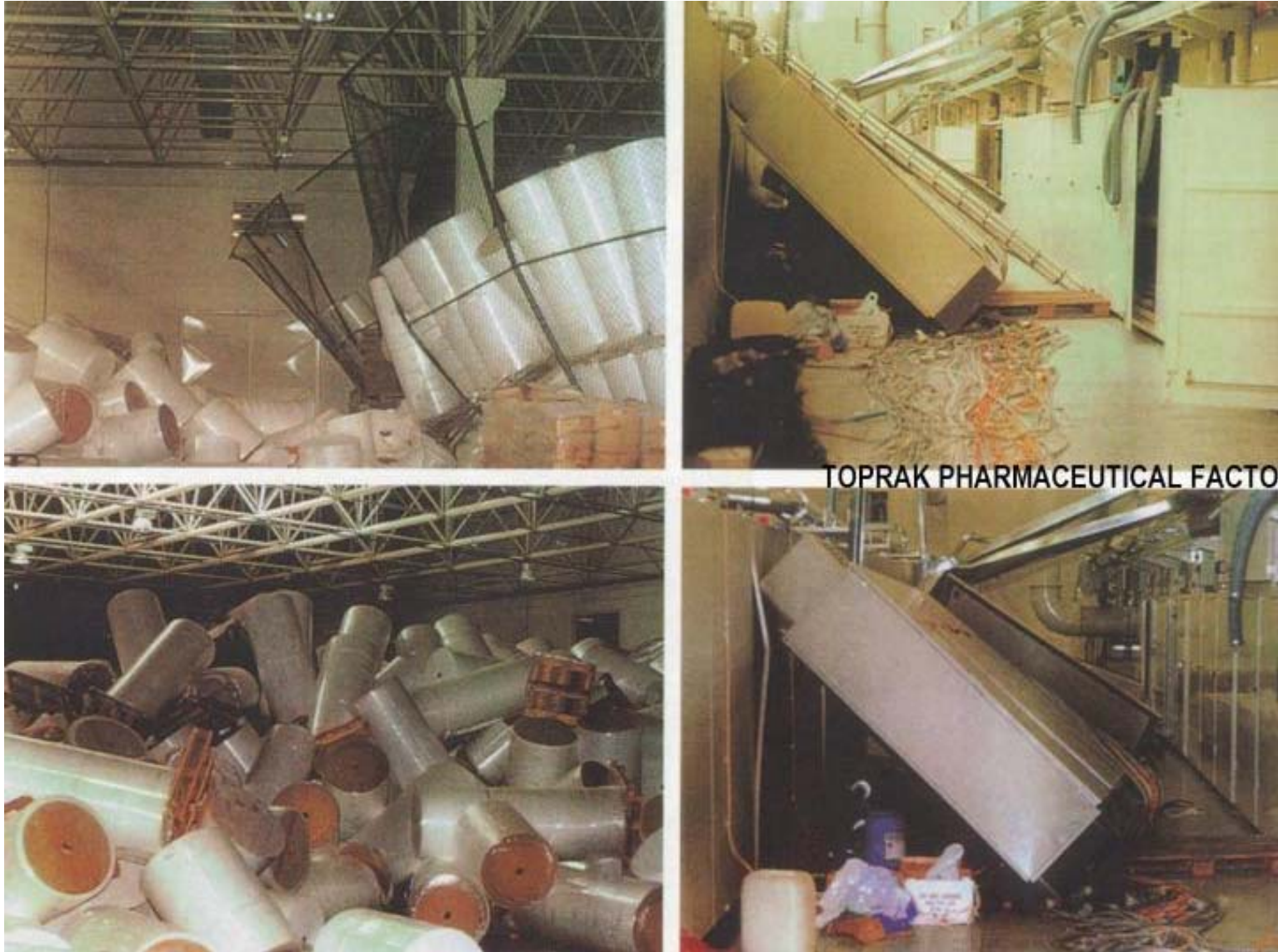
Figure 4.37. Damage at Toprak Pharmaceutical Company (after Milli-Re)
