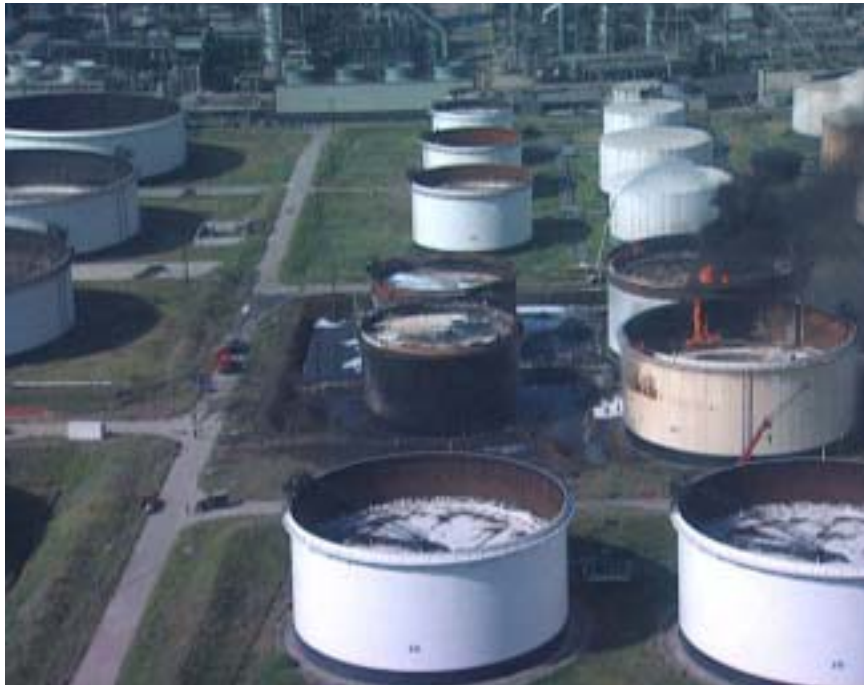
Figure 4.9. Damaged tanks at TUPRAS tank farm.
