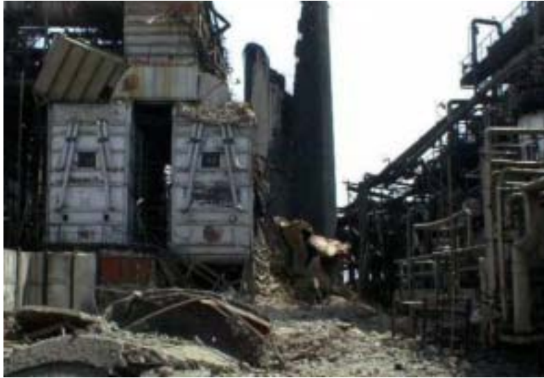
Figure 4.16. Collapsed stack at TÜPRAŞ Refinery.
