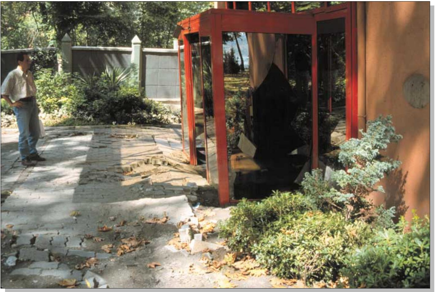
**Figure 38.** Sunken entryway into Sapanca Hotel created when building sank into liquefied soil. *Photograph by Thomas L. Holzer.*
