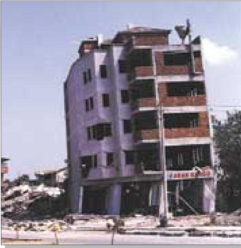
**Figure 43.** Near collapse of building in Adapazari as the result of formation of column hinges in the first story. *Photograph by National Institute of Standards and Technology.*
