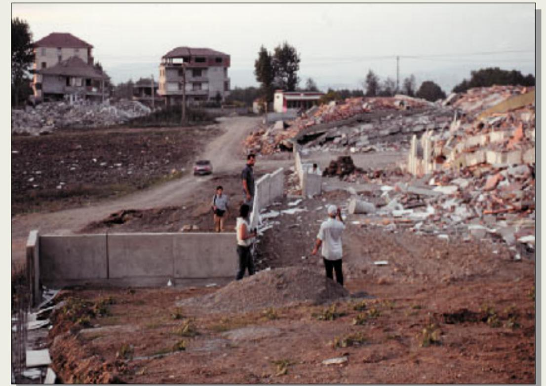
**Figure 15.** Surface rupture extending through boundary wall and collapsed apartments, to the east of Izmit. Strike-slip displacement here was about 3 m. Photograph by Heidi Stenner.
