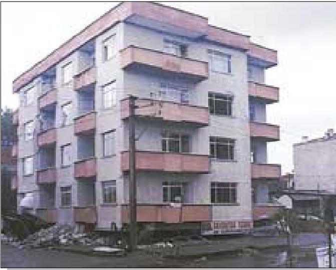
**Figure 41.** Partial building collapse in Yalova as the result of shear failure of first story columns. *Photograph by National Institute of Standards and Technology.*
