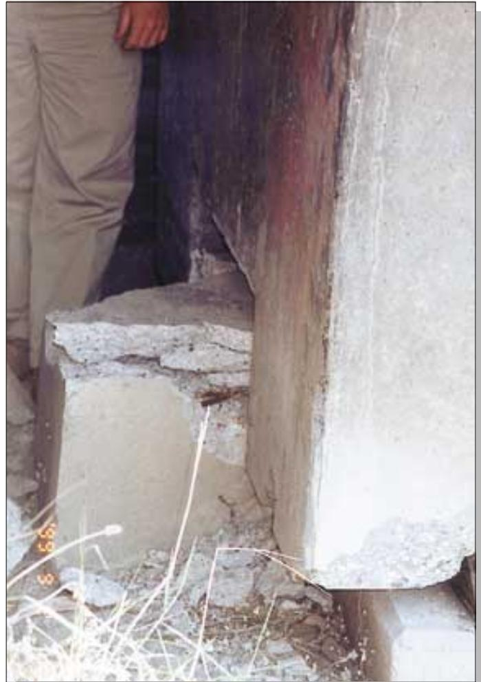
**Figure 50.** Failure of shear keys was common at bridges of the Trans European Motorway. Shear keys at the end of girders prevent transverse and longitudinal seismic movements. *Photograph by Selcuk Toprak.*
