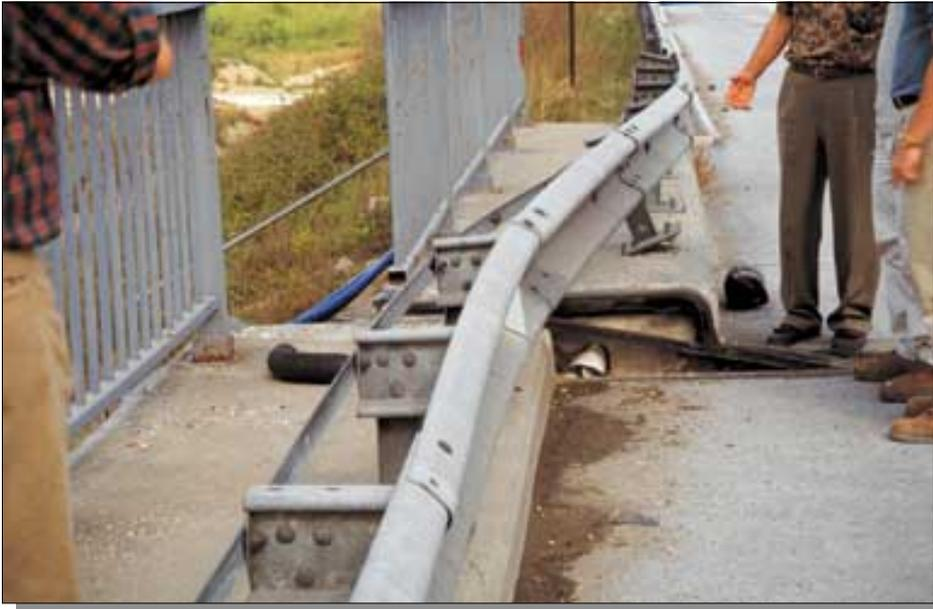
**Figure 51.** Ground shaking caused the westbound span of the Sakarya River bridge to displace 50 cm relative to the east abutment. This was the largest permanent displacement caused by shaking at any bridge. *Photograph by Selcuk Toprak.*
