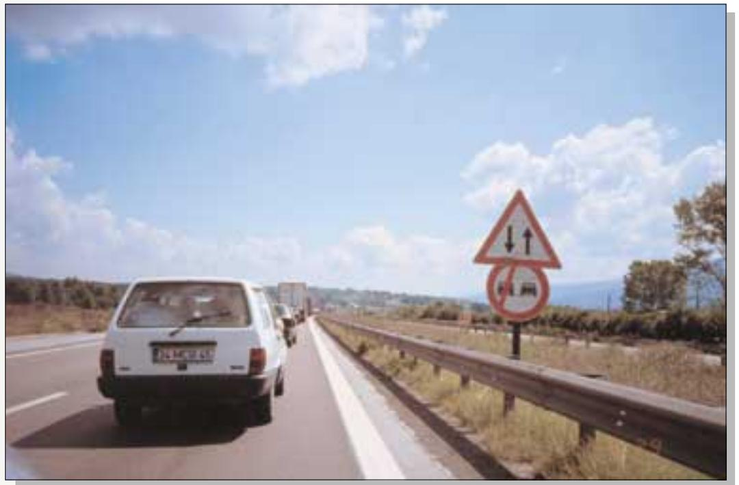
**Figure 48.** Following the earthquake, road surface repairs forced alternative use of the eastbound and westbound lanes of the Trans European Motorway as a two-way highway with greatly reduced speeds from Izmit to about 50 km east of Izmit. *Photograph by Thomas L. Holzer.*
