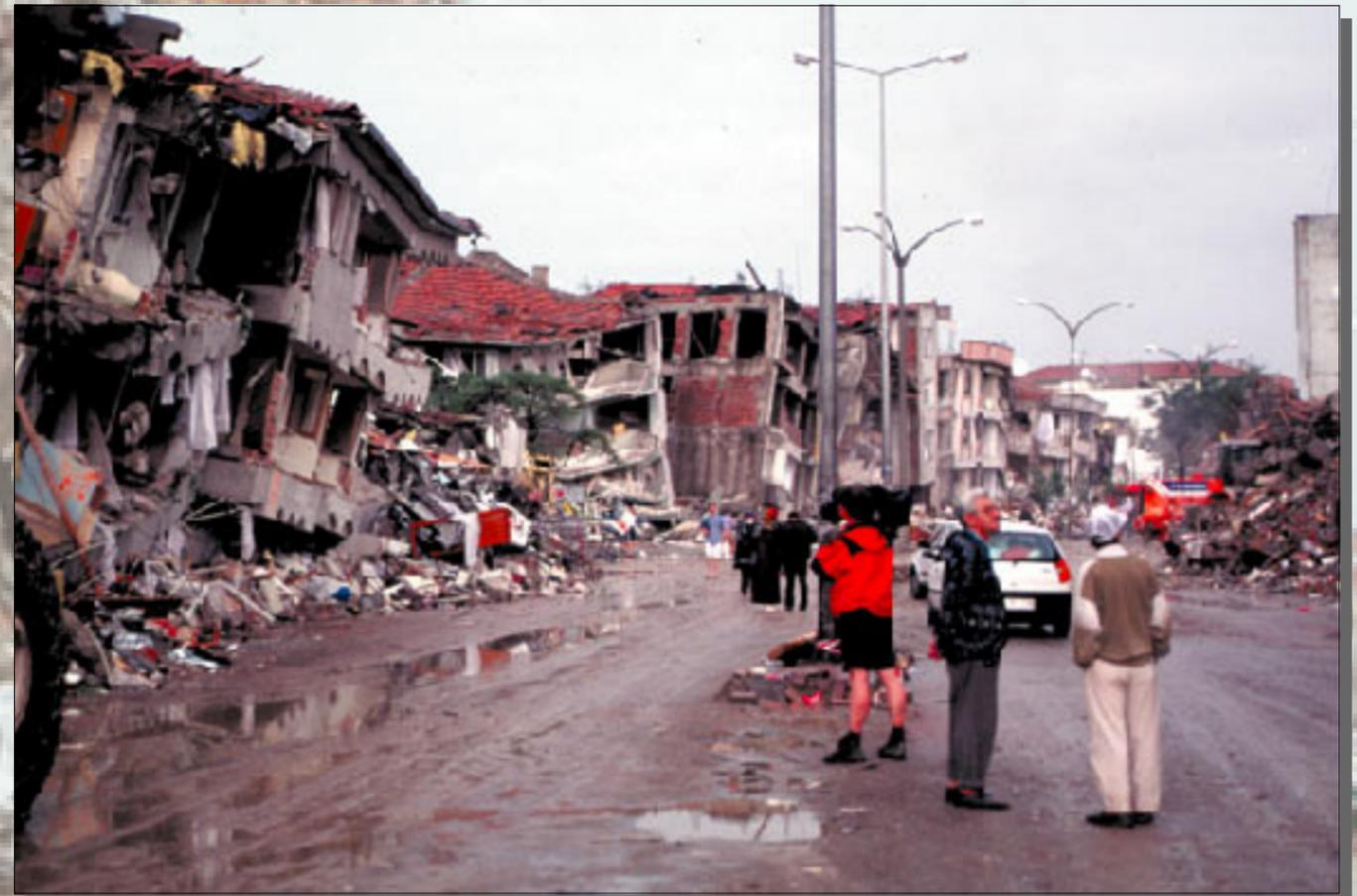
**Figure 57.** Street scene in Adapazari following the Kocaeli, Turkey, earthquake. Extensive damage to concrete structures with little or no ductility displaced more than a quarter of a million people from their homes in the epicentral region. *Photograph by Thomas L. Holzer.*
