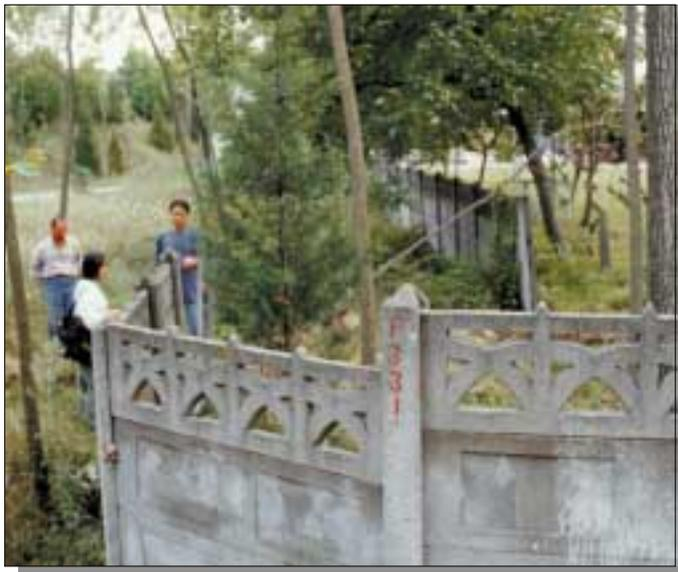
**Figure 18.** Offset wall near Arifiye. The right-lateral displacement is 4.58 m. *Photograph by Heidi Stenner.*
