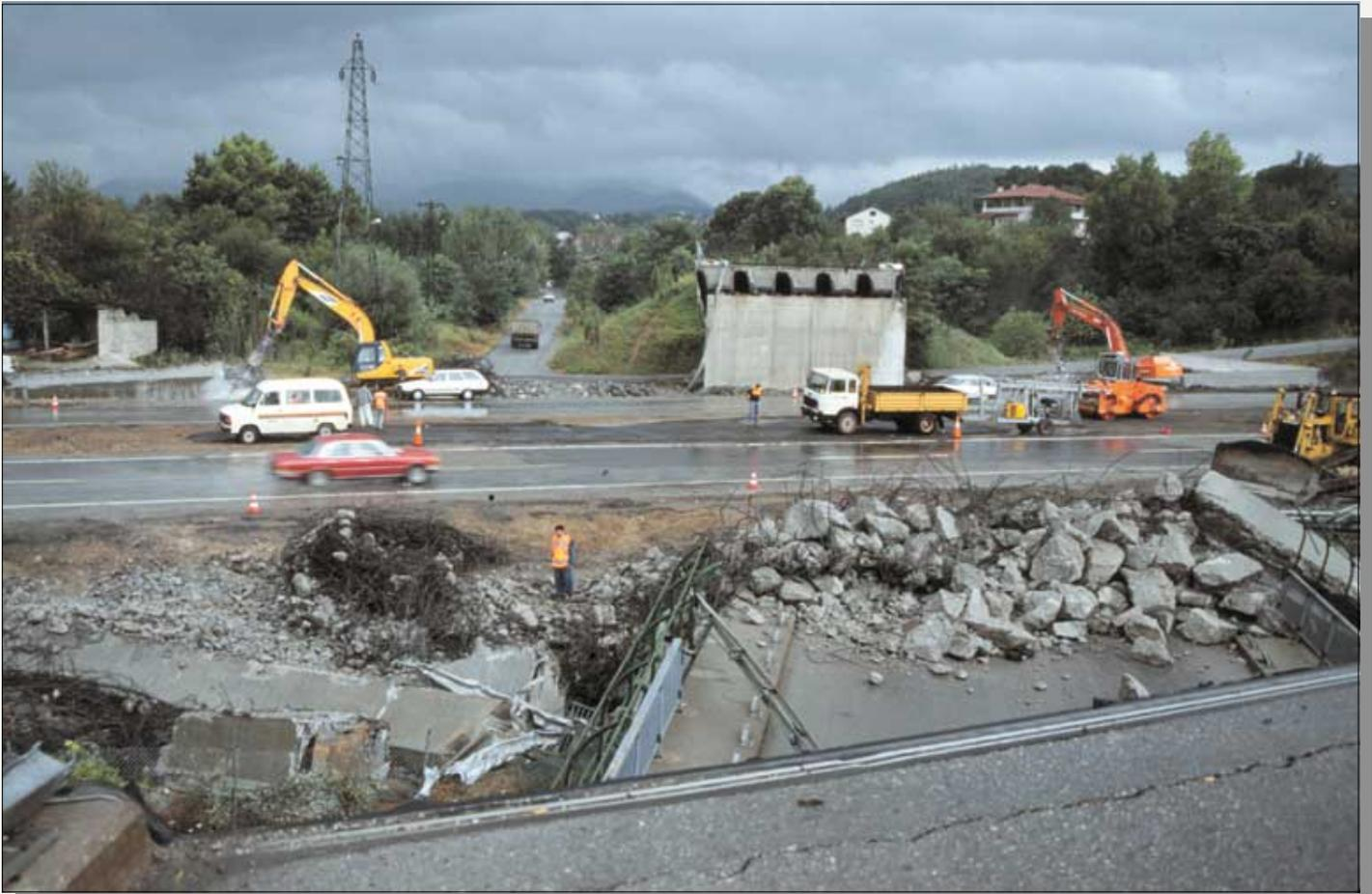
**Figure 53.** The Arifiye overpass collapsed because the surface fault rupture passed directly through its north abutment (foreground). Ten riders of a bus were killed when the bus collided with the collapsed overpass. *Photograph by Thomas L. Holzer.*
