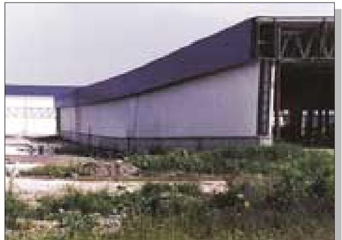
**Figure 45.** Industrial building damaged by near-fault ground movements east of Gölcük. Building is on downthrown block of normal fault and near a major change of strike in the surface fault scarp. *Photograph by National Institute of Standards and Technology.*
