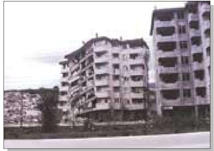
**Figure 42.** Partial collapse of building near Izmit as the result of shear failure of intermediate columns. Note various stages of damage despite apparently similar construction. *Photograph by National Institute of Standards and Technology.*
