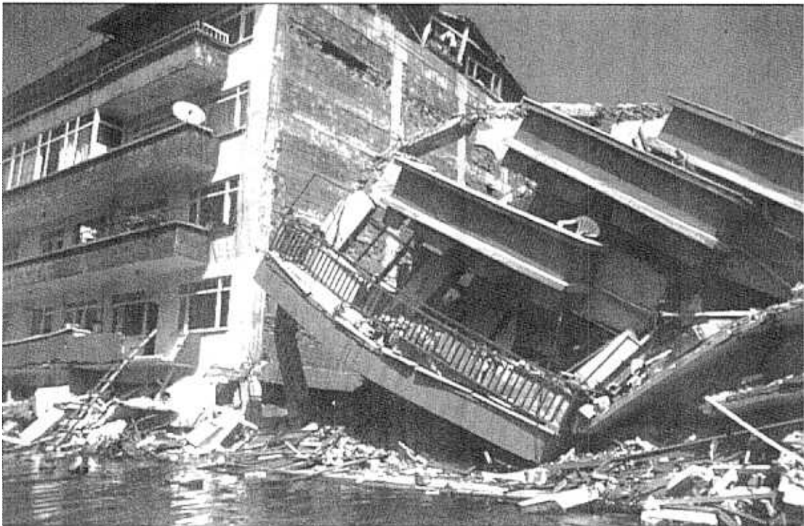
Figure 7 - Inundated buildings in Golcuk. Tectonic displacement along the fault and liquefaction-induced subsidence resulted in extensive areas of flooding along the south shore of Izmit Bay. Note also out-of-plane roof infill, and collapsed building in foreground. (Photo: Aschheim)
