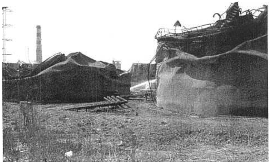
Figure 17 - Tanks destroyed by out-of-control fire in the Tupras refinery tank farm. (Photo: G. Johnson)
