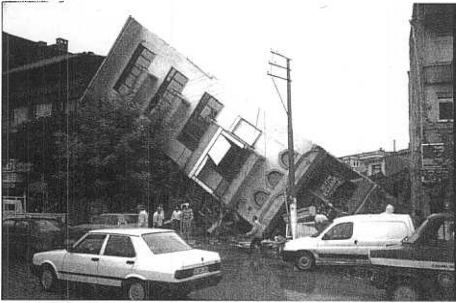
Figure 4 - Building that toppled due to liquefaction-induced loss of bearing strength beneath shallow mat foundation. (Photo: Youd)
