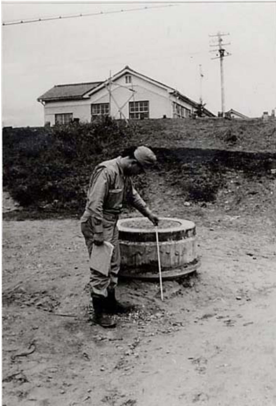
Fig. 5 Uplifted manhole by liquefaction (Near girder bridge of Echigo-line).
