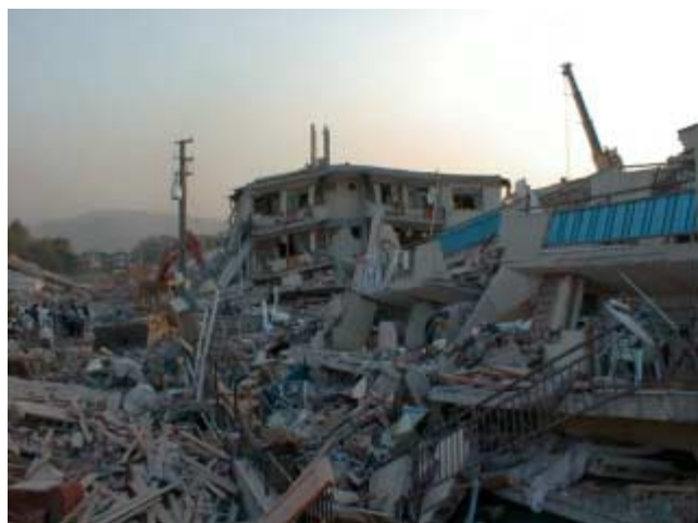
Figure 1. Earthquake damage adjacent to Tupras Refinery, Izmit.
