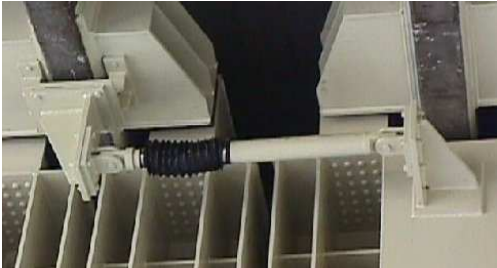
Figure 9.5.6 An example of displacement controlling by damper
