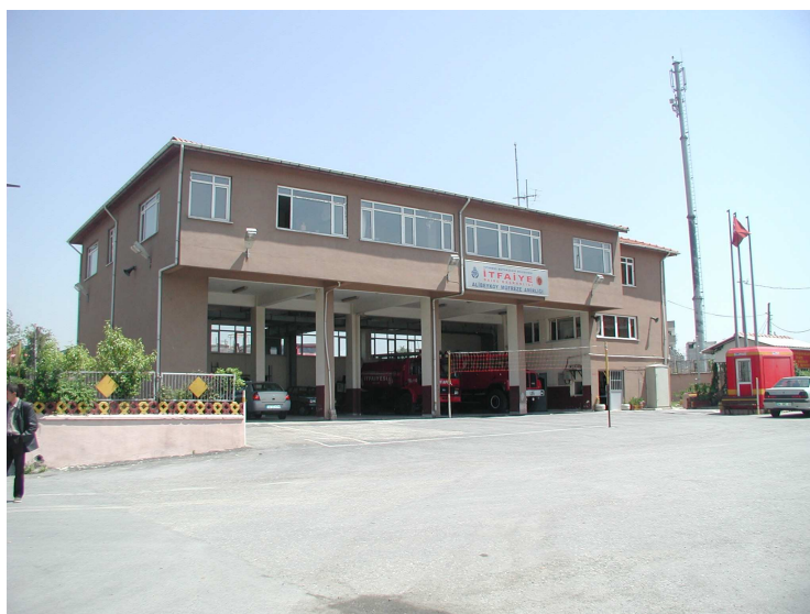
Photo 9.2.2 Fire Fighting Station: Garage and Office within the Same Building
