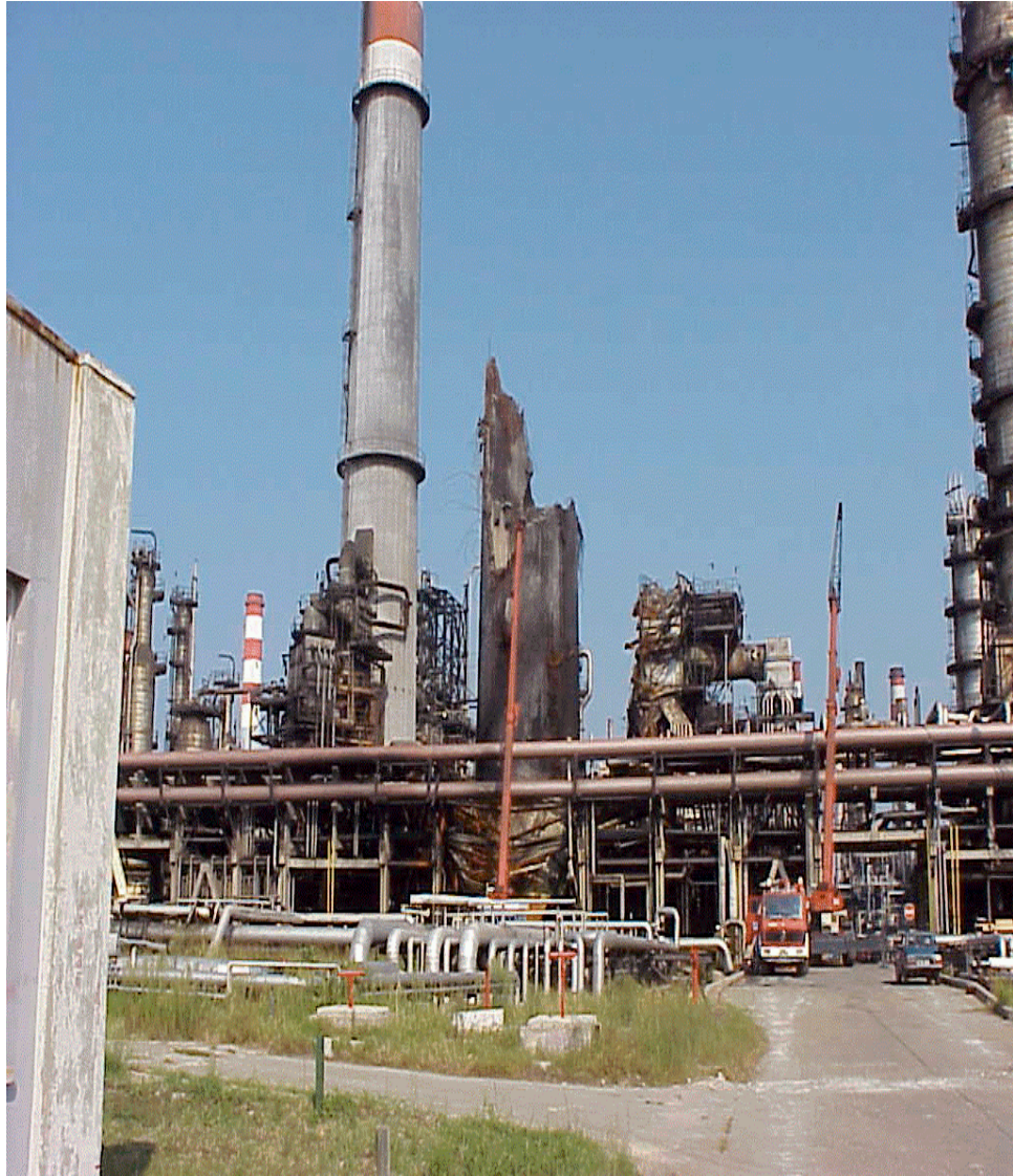
Figure 5: Collapsed 115 m (350') high reinforced concrete stack
