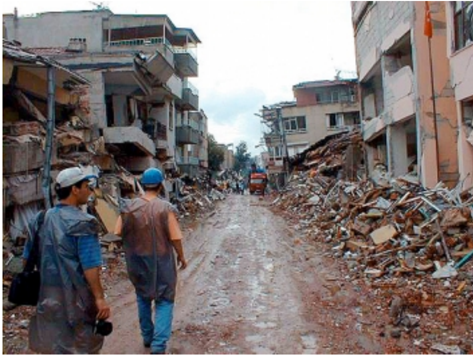
Figure 1: Housing collapses led to thousands of fatalities
