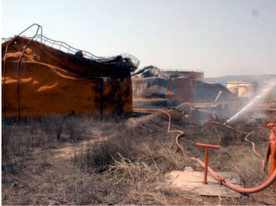
Figure 3: Collapsed tanks in tank farm due to fire
