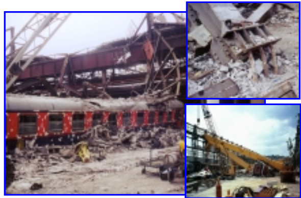
Figure 11: State of damage to wagon factory
