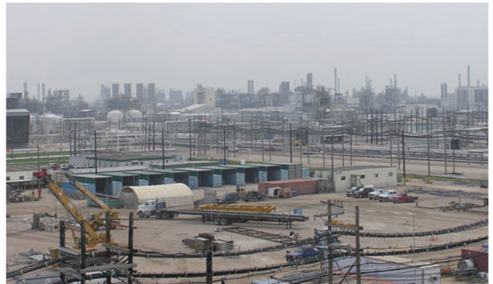
Figure 1. Industrial facilities are complex and individually characteristic
