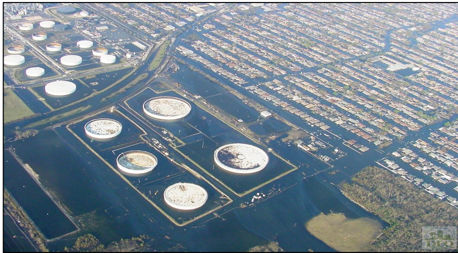
Figure 2. Flood impact in a refinery
