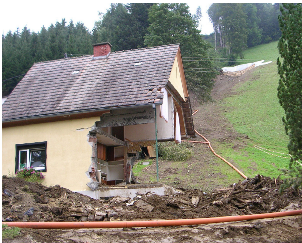
Destroyed house in which two people were killed
