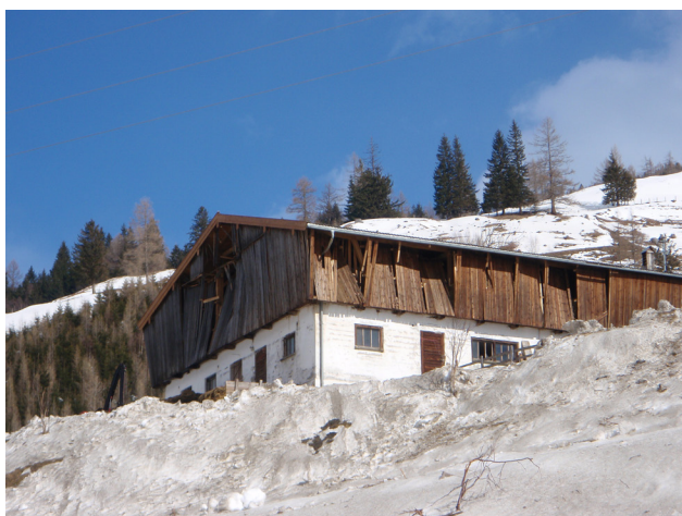
Figure 8.4 Building damaged by the Marchkar avalanche
