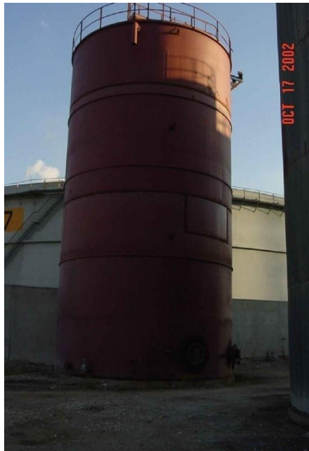
Tank P5151, 24.0m dia., H/D = 0.75, Demin. Water
