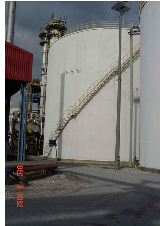
Tank P5151, 24.0m dia., H/D = 0.75, Demin. Water
