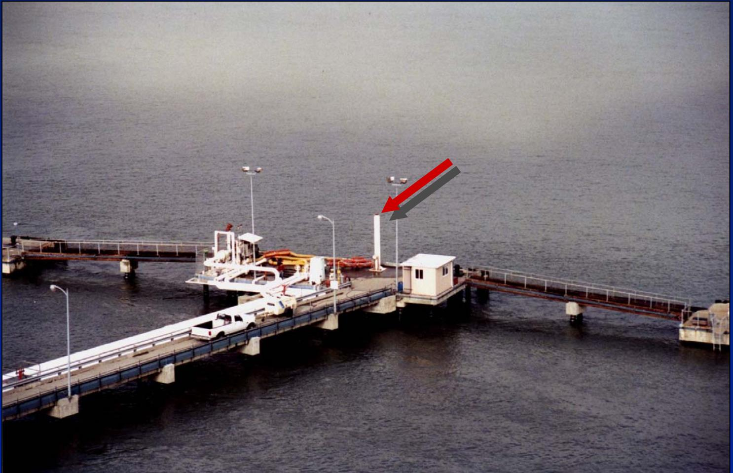
*Broken Loading Arm At Terminal Located in High Current Area*
